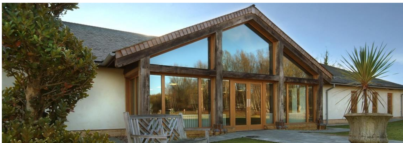
Fig. 4. Sworders' auction rooms, Stansted Mountfitchet, Essex – a single-storey 1100 m 2 building, constructed in 2008 using straw-bale wall construction
